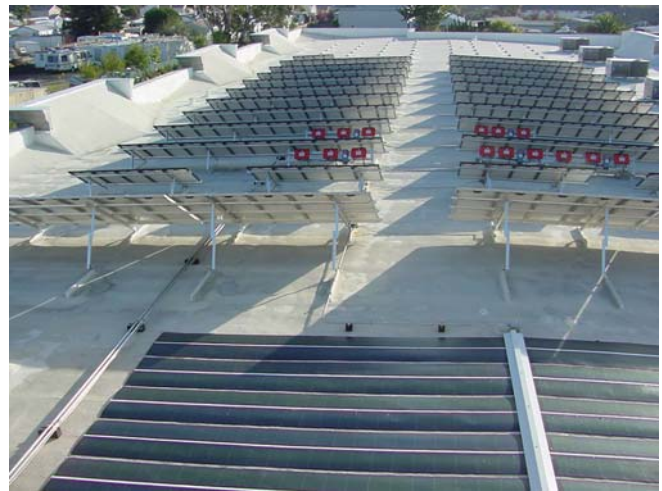
Fig. 1. Three types of solar array: Comparing horizontal amorphous panels, tilted amorphous panels and polycrystalline panels
