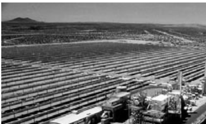
Fig. 14a: A portion of the world’s largest solar thermal-electric generator (on the left), part of the 354 MW system in California. Shown also is the embedded gas-fired generator for 25 % “hybrid” operation, to level the output of the solar system, demonstrating a useful synergy between renewable energy and conventional energy production.
