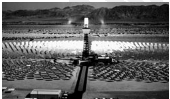
Fig. 14b: Solar I, the 10MW “power tower” in southern California. Source Fig. 14a: NREL Source Fig. 14b: U.S.D.O.E.
