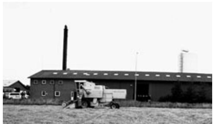
Fig. 6b: Community combined heat and power (CHP) plant, fueled by waste straw grown in the near vicinity, for 300 families in Denmark Photograph by Dr. Donald Aitken
