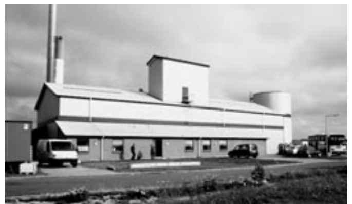
Fig. 5b: Community combined heat and power (CHP) plant, fueled by wood chips, for 300 families in Denmark Photograph by Dr. Donald Aitken
