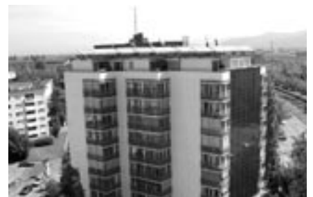
Fig. 16b: A multifamily building in Freiburg, Germany, using the roof for solar water heating, and the south wall for solar electric energy production.
