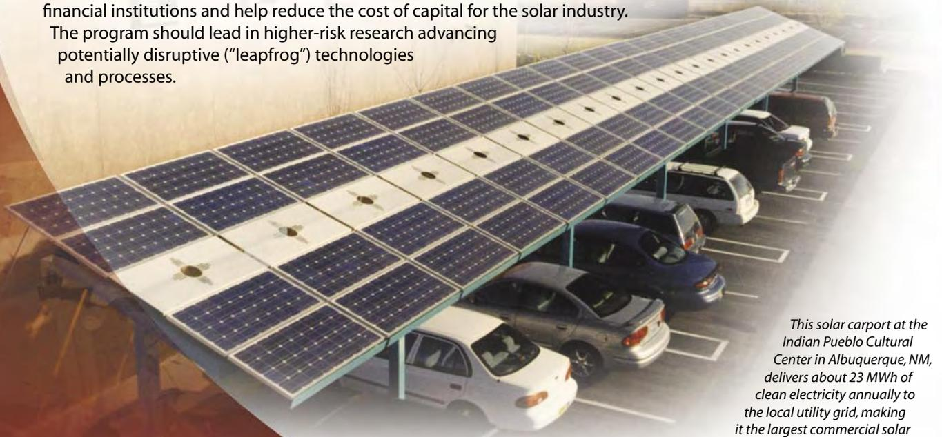
*This solar carport at the Indian Pueblo Cultural Center in Albuquerque, NM, delivers about 23 MWh of clean electricity annually to the local utility grid, making it the largest commercial solar power system in New Mexico. (credit: Sandia National Laboratories)*
